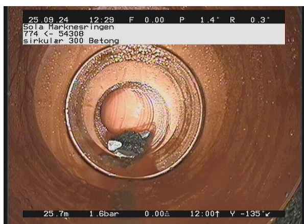
Marknesringen_774_55638.jpg, 00:07:15, 25.78m Materialendring. Plast
